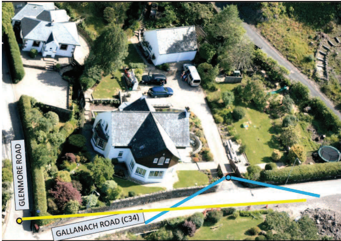
Figure 3: Aerial view of The Carding Mill showing visibility splays from proposed altered gateway to the property (in blue) and the potential enhanced visibility from Glenmore Road onto Gallanach Road (in yellow) that could be created.
