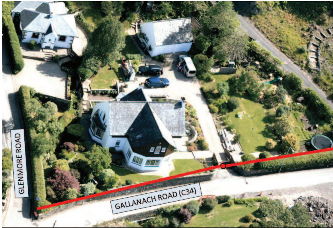
Figure 1: Aerial photo of The Carding Mill, showing the entrance with the requested visibility splays marked in red. The splay to the left cuts through a stone wall in front of the house and the splay to the right will require removal of the beech hedge. The children's play area can be seen to the right of the site.
